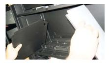
Orient the stainless side panels with the larger fold in the panel facing in towards the burner and facing the back of the firehox
